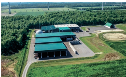
Biomassevergärungsanlage (BMV) in Dörpen
